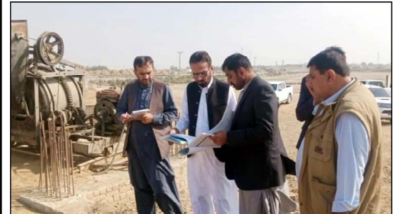
SOHBAHPUR: Member Chief Minister Inspection Committee Aslam Tareen being briefed by XEN Ahmed Nawaz Umrani about under construction projects
