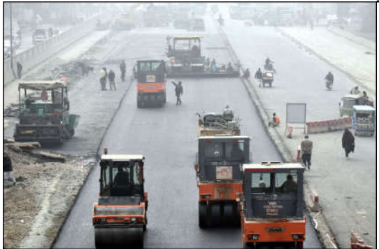
LAHORE: Labourers are busy in construction work of Sagian Road with the help of heavy machinery in the Provincial Capital.
