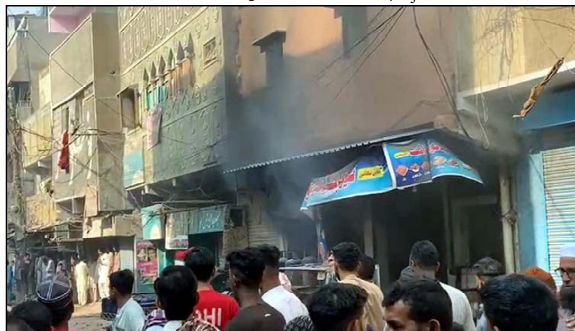
KARACHI: View of damages after gas cylinder blast occurred at gas cylinder filling shop while rescue operation and investigation is underway, at Keamari KPT Gate No 15 nearby Khushboo Center in Karachi.
