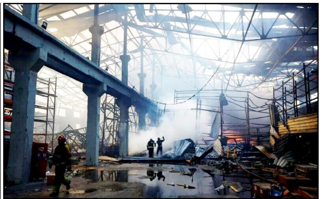
Rescuers work at the site where a residential building was damaged during a Russian missile and drone strike, amid Russia's attack on Ukraine, in Odesa, Ukraine
