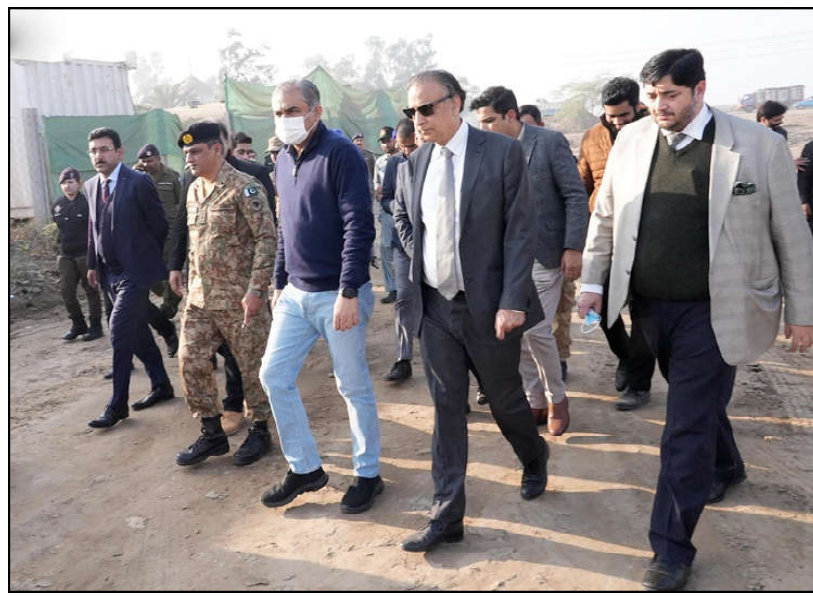
LAHORE: Caretaker Chief Minister Punjab Mohsin Naqvi inspecting the under construction work of Lahore Ring Road Southern Loop-III Project.
