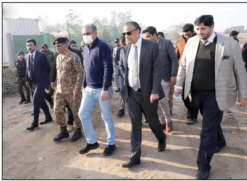
LAHORE: Caretaker Chief Minister Punjab Mohsin Naqvi inspecting the under construction work of Lahore Ring Road Southern Loop-III Project.
