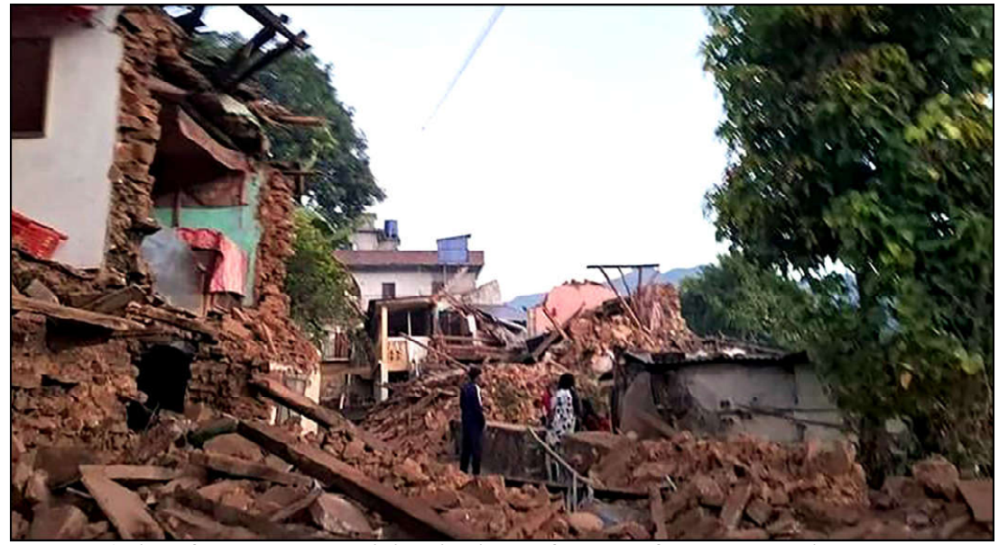
A view of damaged houses lie in ruins, in the aftermath of an earthquake in Nepal.
