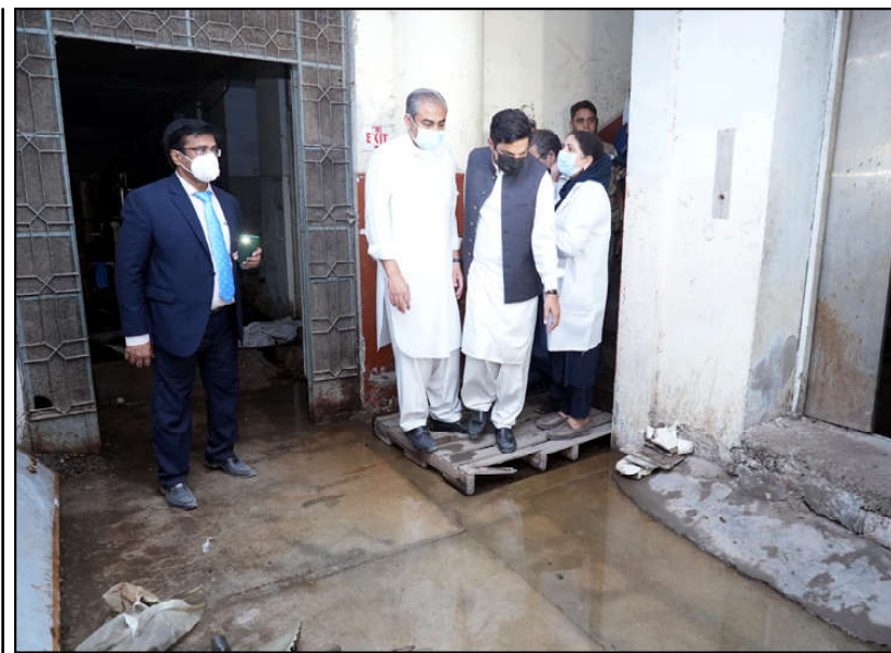
LAHORE: Caretaker Chief Minister Punjab Mohsin Naqvi giving direction regarding standing water in basement of Services Hospital during his visit.
