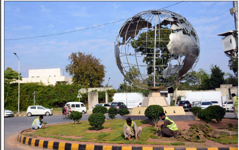
ISLAMABAD: Workers of Capital Development Authority (CDA) is installing artificial green grass alongside Constitution Avenue in Federal Capital.
