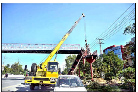
ISLAMABAD: Labourers busy in installing new pedestrian bridge at IJP Road.
