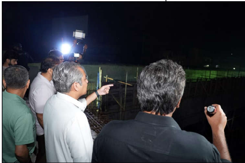
LAHORE: Caretaker Chief Minister Punjab Mohsin Naqvi inspecting construction of Shahdara Flyover project.
