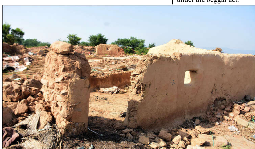
ISLAMABAD: A view of demolished houses during Islamabad Police and Capital Development Authority (CDA) joint anti-encroachments operation of illegal Afghan Basti, in Federal Capital.
