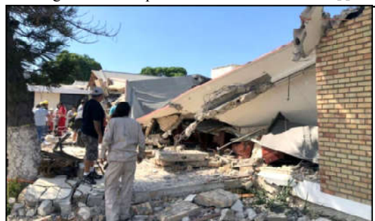
Members of a rescue team and people work at a site where a church roof collapsed during Sunday mass in Ciudad Madero, in Tamaulipas state, Mexico in this handout picture distributed.
