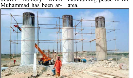
HUB: Construction works of Sindh and Balochistan connecting Bridge is underway, in Hub.
