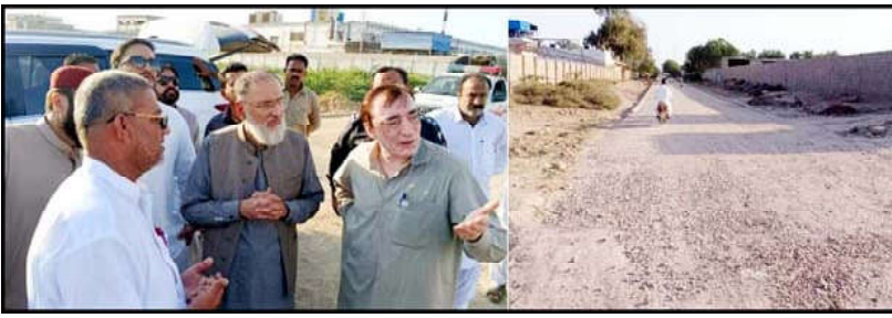
HUB: Caretaker Provincial Minister for Industries, Excise and Taxation Prince Ahmed Ali Ahmedzai issuing directives to M/LIEDA during his visit to site of under construction road network project
