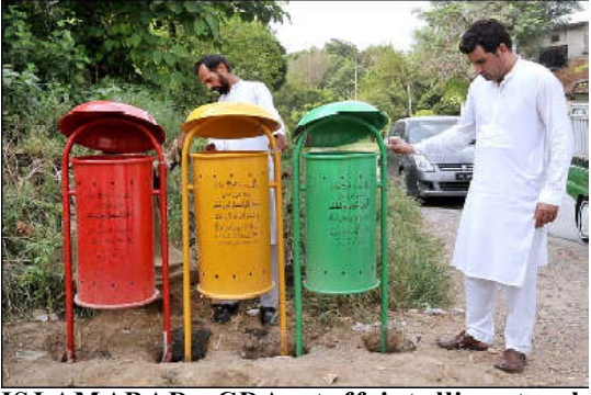
ISLAMABAD: CDA staff installing trash containers along the roadside.
