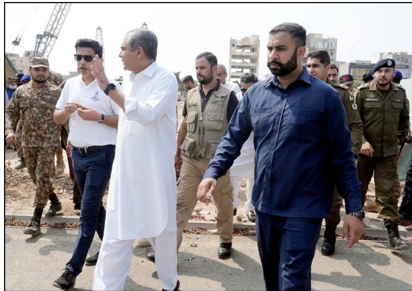
LAHORE: Caretaker Chief Minister Mohsin Naqvi giving directives during inspecting of earth work of Ring road passing from Bahria Town under Loop Three project.
