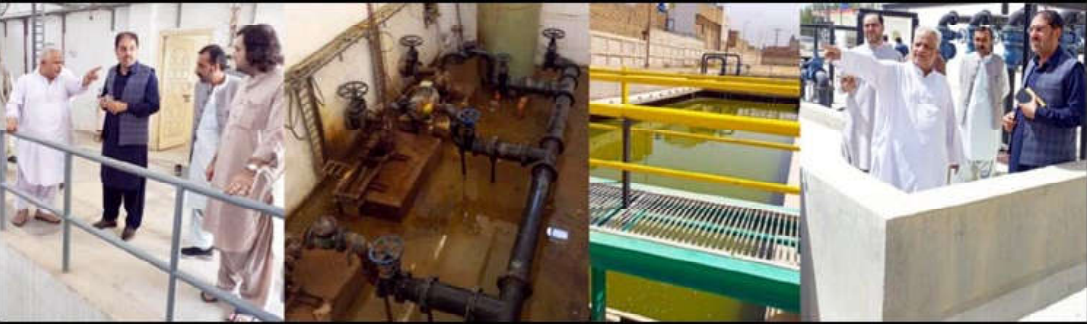
QUETTA: Caretaker Provincial Minister for PHE & Population Welfare Sardar Ejaz Ahmed Khan Jaffar inspecting water treatment plant and booster pump at Sabzal road.
