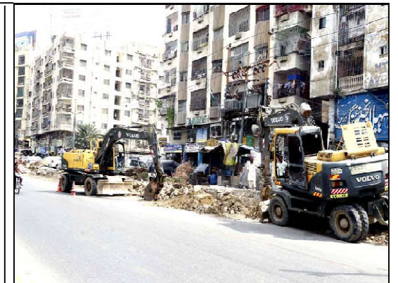
KARACHI: Construction works of new development projects for extending road is underway under the supervision of local government department, as slow pace of construction work is creating problems for commuters due to traffic jam and they demand to concerned department to complete work as soon as possible, located on Shahrah-e-Faisal road in Karachi.
