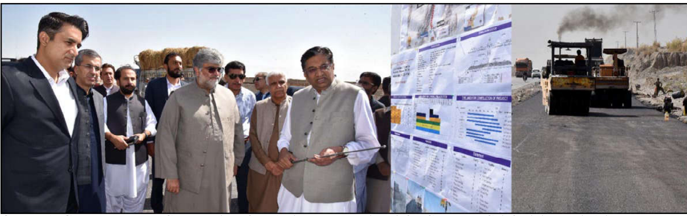
QUETTA: General Manager Construction of NHA Bisharat Hussain briefed Caretaker Chief Minister Mir Ali Mardan Khan Domki
