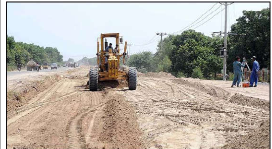
MULTAN: Head Muhammad Road is currently undergoing expansion to ensure smoother traffic flow. This vital route connects several cities in South Punjab, Balochistan, and Khyber Pakhtunkhwa (KPK).
