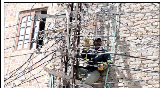
HYDERABAD: HESCO workers busy in disconnection of illegal connections in Latifabad.
