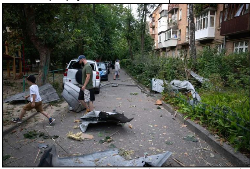
Local residents pass by debris that fell down from their damaged house after a Russian rocket attack in Kyiv, Ukraine.
