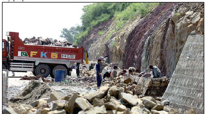
ISLAMABAD: Labourers busy in building a boundary wall on Islamabad Expressway.
