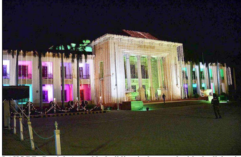
LAHORE: Punjab Assembly building is decorated with the lights in celebration of Independence Day
