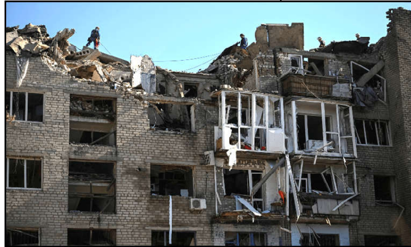
Rescuers work at a site of a building destroyed during a Russian missile strike, amid Russia's attack on Ukraine, in Pokrovsk, Donetsk region, Ukraine.
