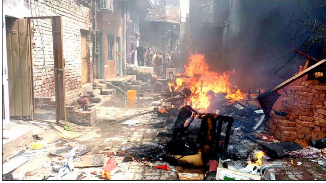
FAISALABAD: View of site after a mob enraged over blasphemy allegations set on fire several churches and a number of houses belonging to Christians in Jaranwala tehsil of Faisalabad.
