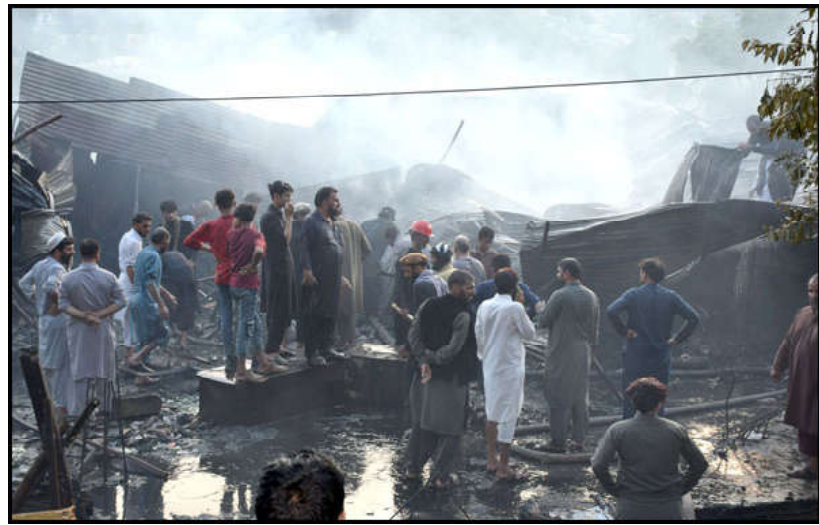
MUZAFFERABAD: A destructive view of the warehouse as burnt after fire due to short circuit, near Tanga stop at the Capital of AJK.
