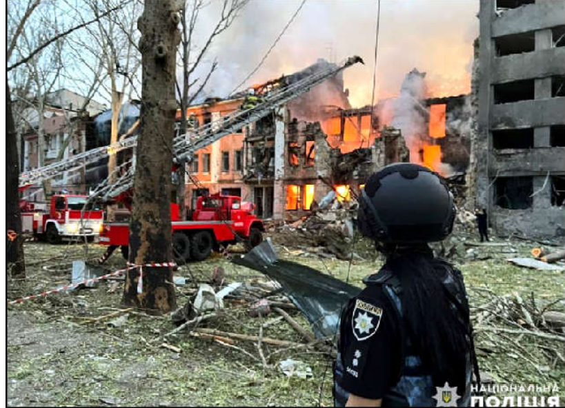
Emergency services personnel work at the site of a building that was damaged by a Russian missile strike, amid Russia's invasion of Ukraine.
