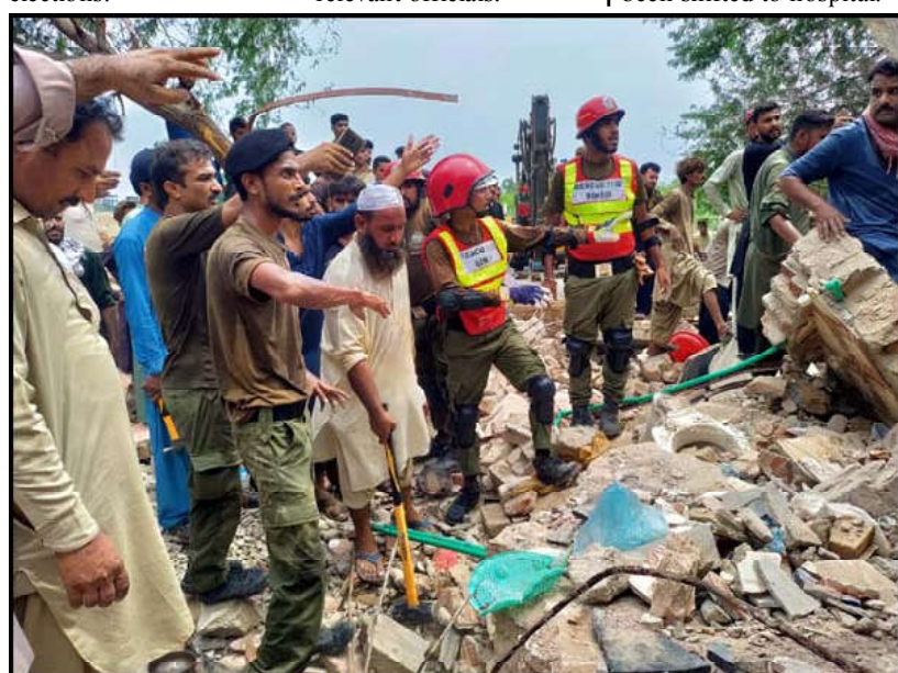
SUKKUR: Rescue officials are busy in rescue operation after a two-storey building collapsed due to heavy rainfall, in Sukkur on Monday, July 24, 2023. Four people were dead and several others were injured as a two-storey building collapsed in Sukkur due to heavy rainfall on Monday.
