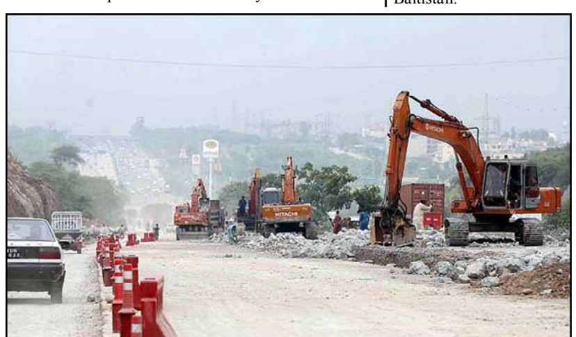
ISLAMABAD: Heavy machinery being used to build new lanes on Islamabad Expressway.
