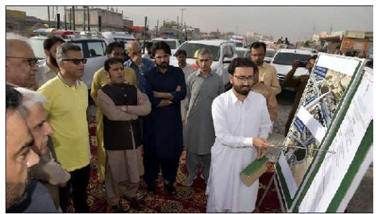
QUETTA: Chief Secretary Balochistan Abdul Aziz Uqaili being briefed about under construction Gai Khan Chowk Flyover project
