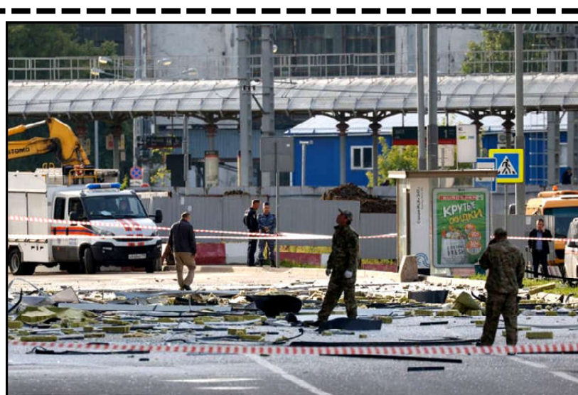
Members of the security services investigate the site of a damaged building following a reported drone attack in Moscow, Russia.
