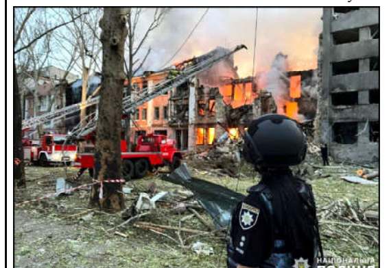
Emergency services personnel work at the site of a building that was damaged by a Russian missile strike, amid Russia's invasion of Ukraine.
