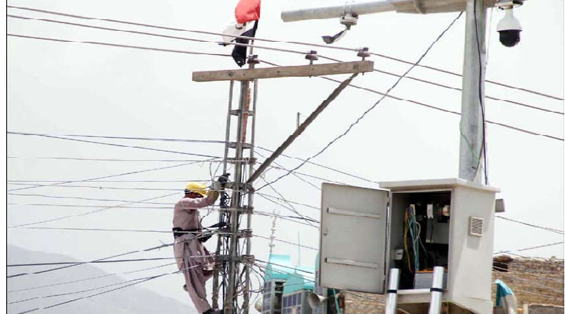
QUETTA: Technician is busy in maintenance works of CCTV camera in connection of Shiite religious mourning procession in memories of martyrdom of Hazrat Imam Hussain (RA), grandson of Prophet Mohammad (PBUH), on the route of Ashura Procession.
