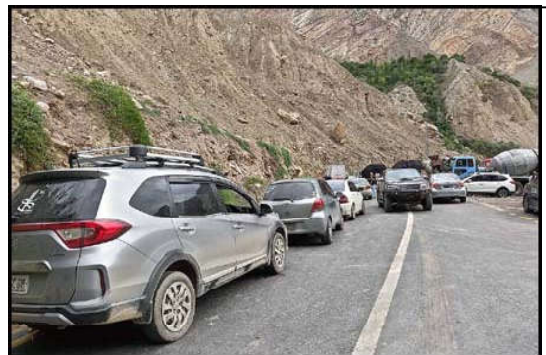
GILGIT: Massive traffic jam after land sliding near Shingus Paari at Juglot-Skardu Road (JSR).
