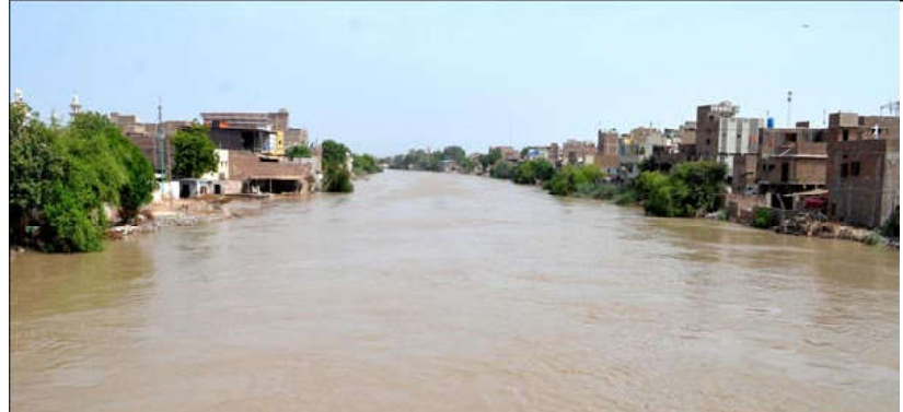
HYDERABAD: View of the water level increasing in the Phuleli Canal while many nearby residents evacuate from their homes due to increased water level and overflowing canal water, in Hyderabad.
