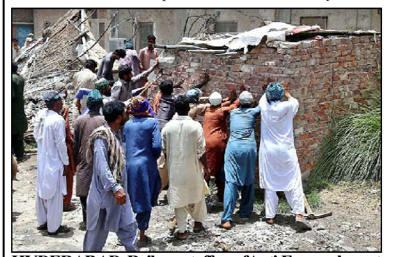
HYDERABAD: Railway staffers of Anti-Encroachment Cell demolishing encroachments at Makkhi Shah area.
