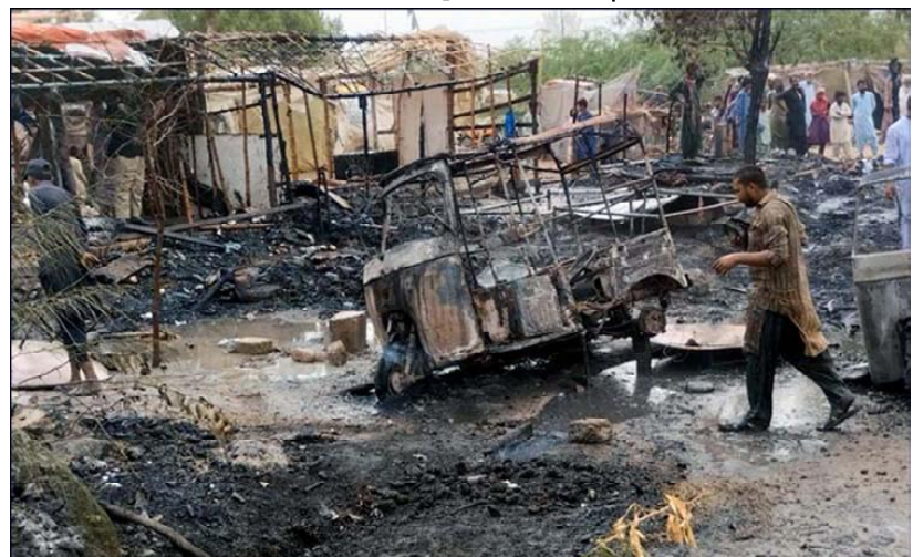
KARACHI: View of site after fire eruption incident in a slum due to unknown reasons, while residents restored their makeshift houses, at Super Highway road nearby Jamali Bridge.
