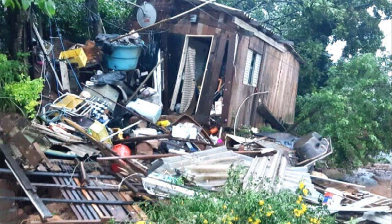
View of a house destroyed in the city of Sao Leopoldo, Rio Grande do Sul State, after an extratropical cyclone hit the southern region of Brazil, causing thunderstorms and windstorms.
