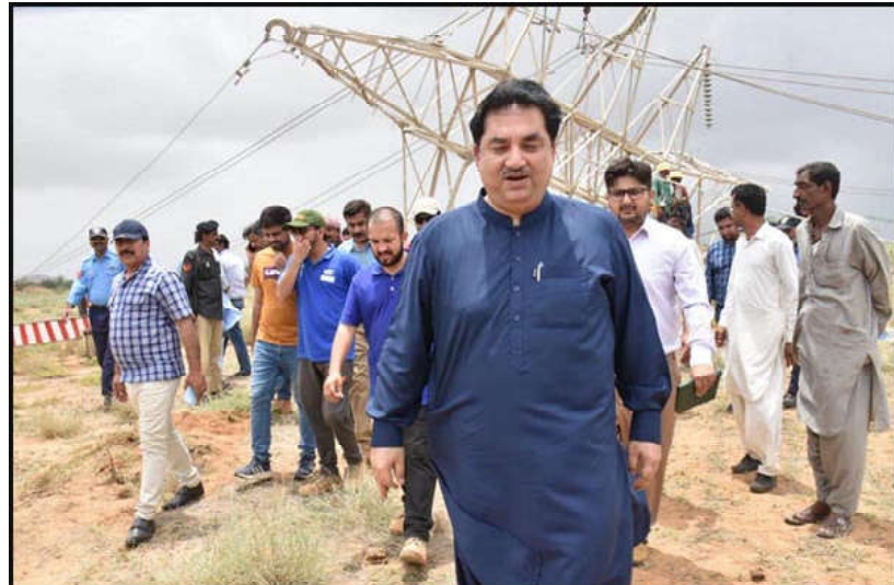
JHAMPIR: Engineer Khurram Dastagir, Federal Minister for Power visiting the damaged towers of Wind Power Projects due to recent cyclonic wind.
