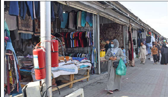
ISLAMABAD: A view of fire extinguisher install bed shop keeper outside his shop at H-9 Sunday Bazar as after fire in weekly Sunday Bazar shop-keepers are taking care by their own.
