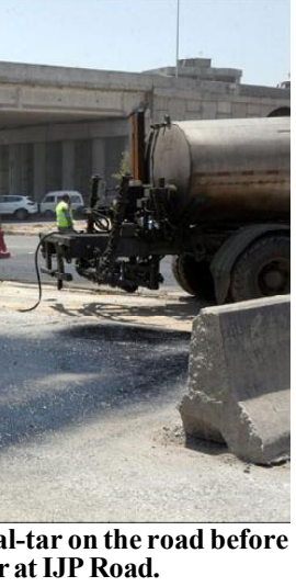
ISLAMABAD: Laborers are busy in spraying Coal-tar on the road before carpeting the patch under newly constructed flyover at IJP Road.
