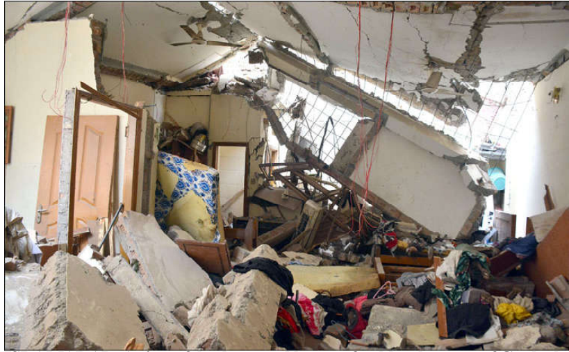
ISLAMABAD: A view of the destroyed house after blast because of Gas leakage at Peoples Colony in City.
